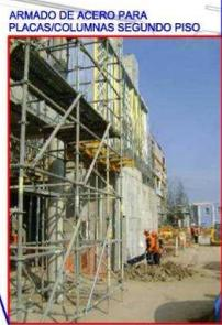
ARMADO DE ACERO PARA PLACAS/COLUMNAS SEGUNDO PISO
