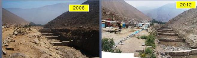
The slide shows two side-by-side photographs of spillway dikes. The left photo is labeled '2008' and shows a clear, functional dike. The right photo is labeled '2012' and shows the same dike heavily silted up with sediment, significantly reducing its height and effectiveness.
